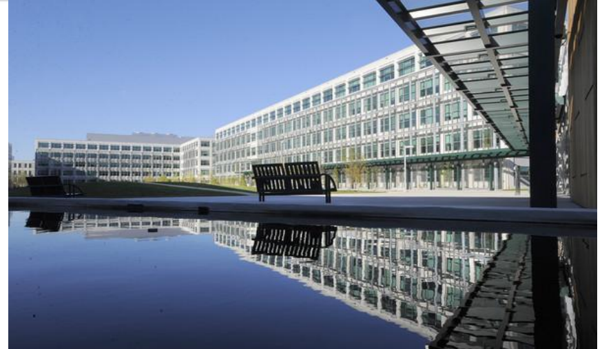
New Team C4ISR Buildings
