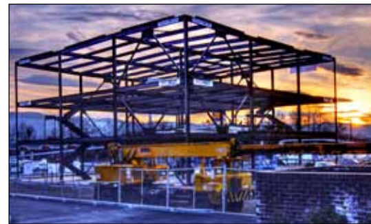
Barnett branch construction underway.
