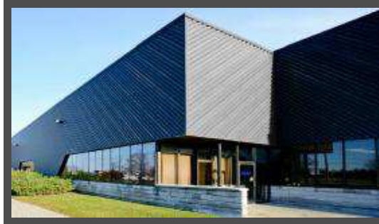
296-300 Walker Drive, Brampton
