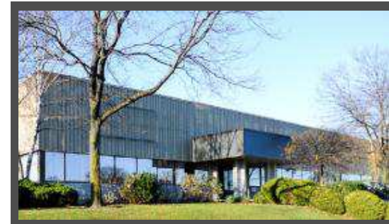
6 Shaftsbury Lane, Brampton
